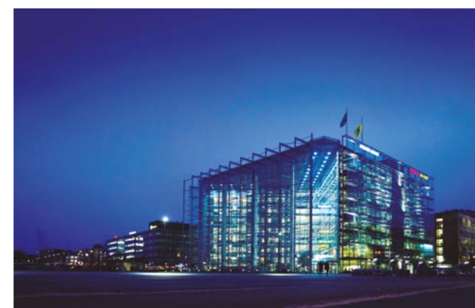
Commercial and Office Building - HELSINKI (FINLAND) • Area: 38.190 m2; Built: 1999 • Open and distributed spaces, 1.400 people working daily, scheduled occupancy
